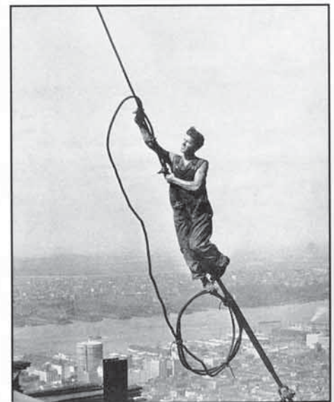
▲ Copyright reproduced from the Collections of Library of Congress Lewis Wickes Hine Carpentieri sull'Empire State Building 1931
